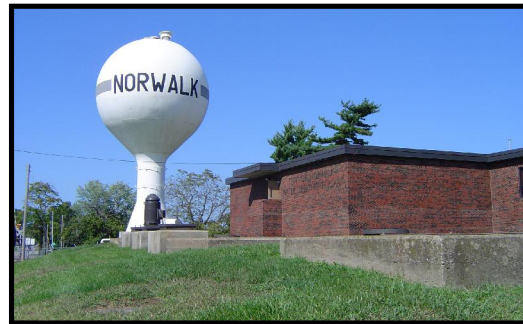
Norwalk's water treatment plant
