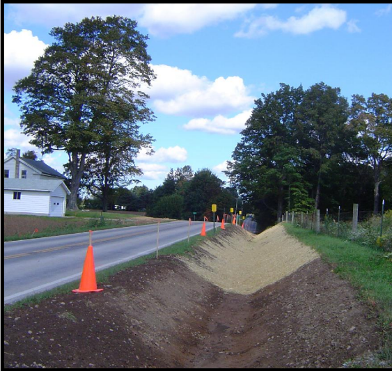
Ditch improvements along Ridge Road south of Norwalk
