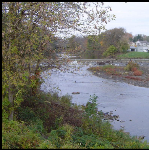
View of the Huron River dam in Monroeville
